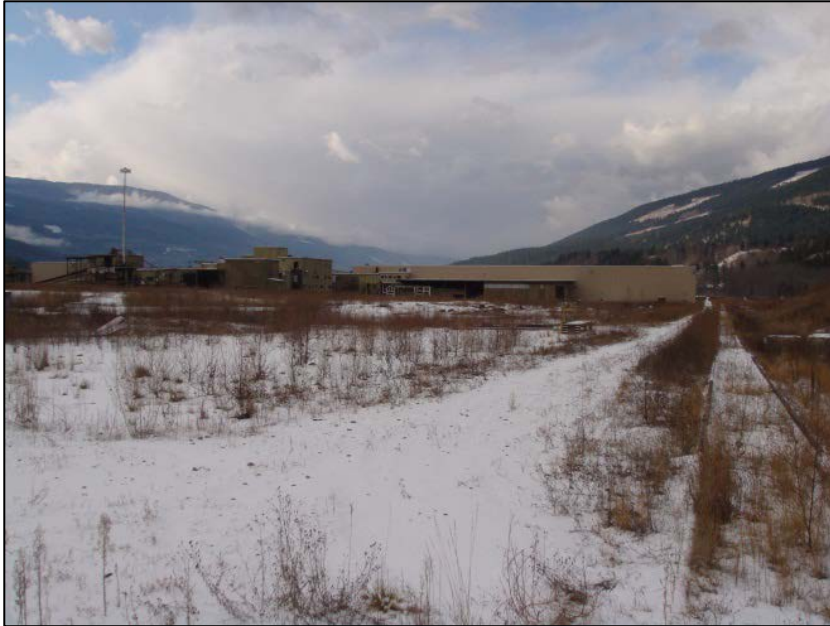
Figure 18-5: Rail Siding West to Old Mill Building
