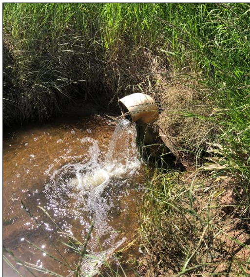
Photo 2. Water control structure outflow.
